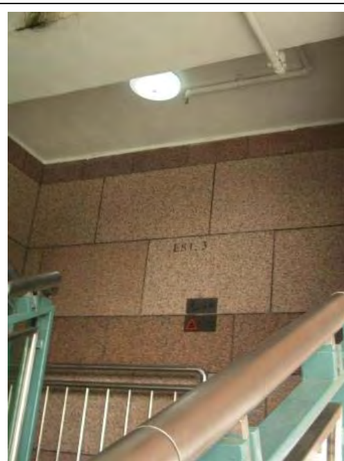
LED Circular Tube c/w PIR sensor Installed at EST 3 staircase
